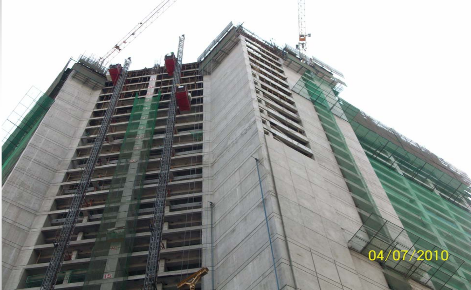
North elevation of the building
