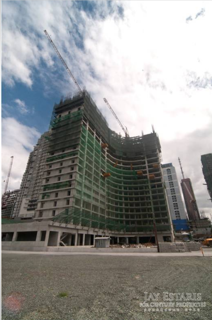
At 22 floors in January
