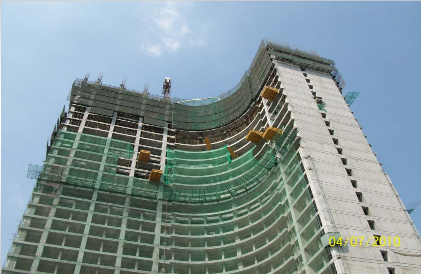
South elevation of the building
